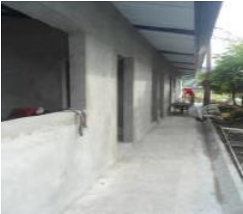
Avance general frente Caniles.
